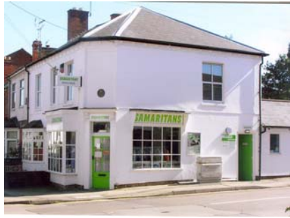
Left: The Earlsdon Cottage (15)
