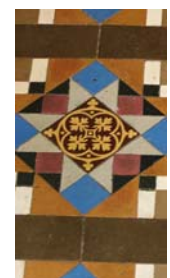
Arden Street Porch floor tiles
